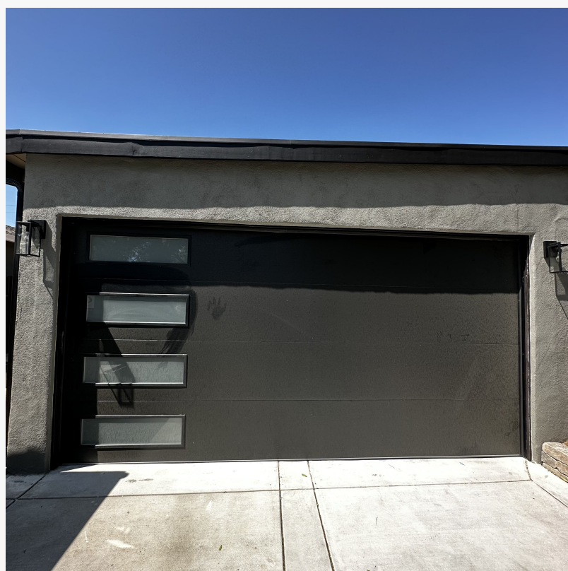
commercial garage door repair
