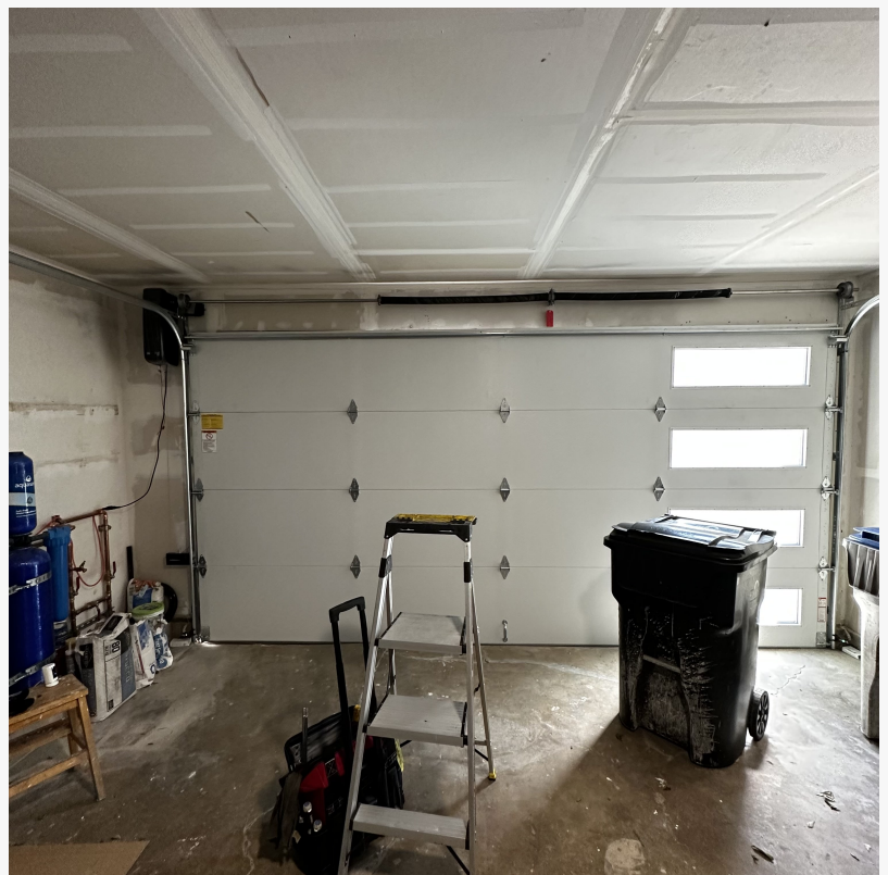
garage door inspections
