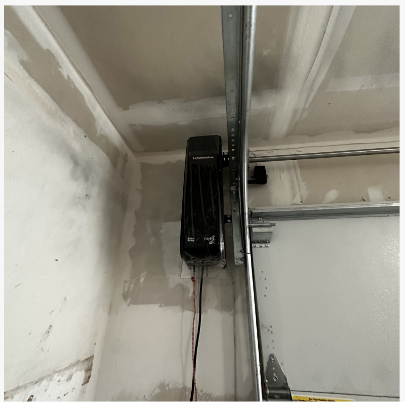
emergency garage door repair
