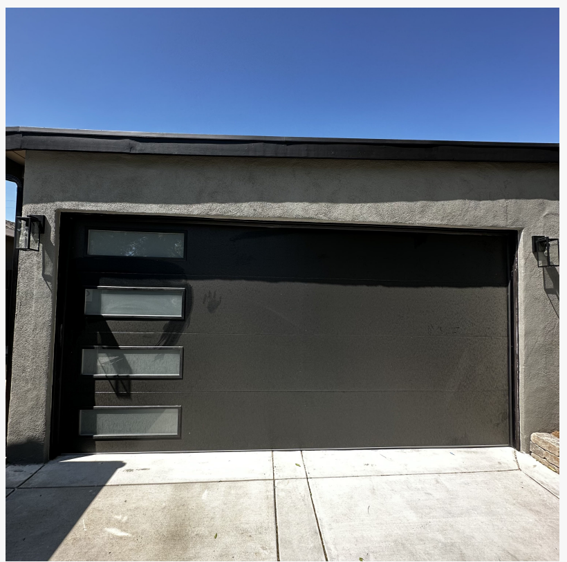
emergency garage door repairs
