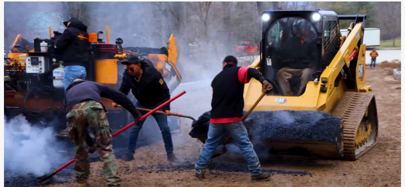
Asphalt Parking Lot Installation
