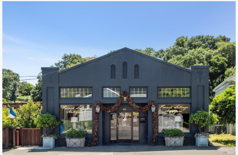
Exterior of 303-307 Bodega Ave, Petaluma, CA
