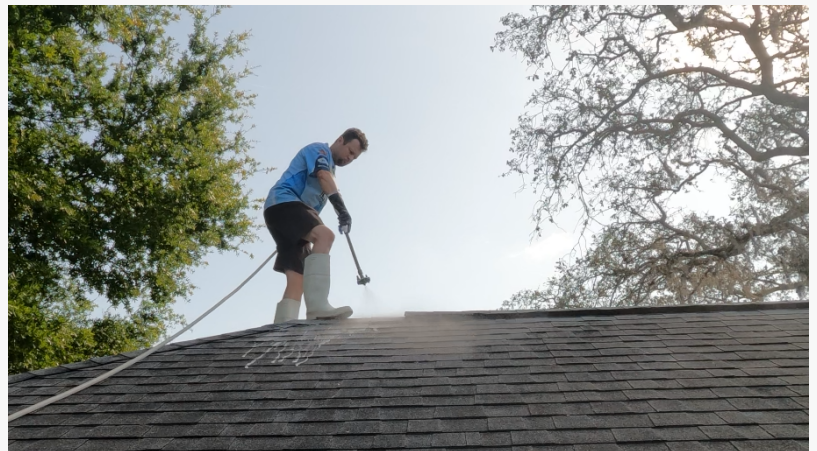
Roof Washing Central Florida Community Home
