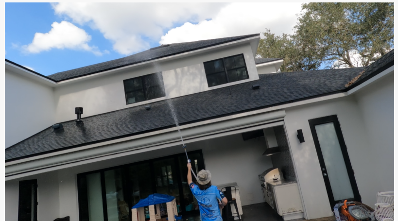
Soft Washing Roof Cleaning Central Florida
