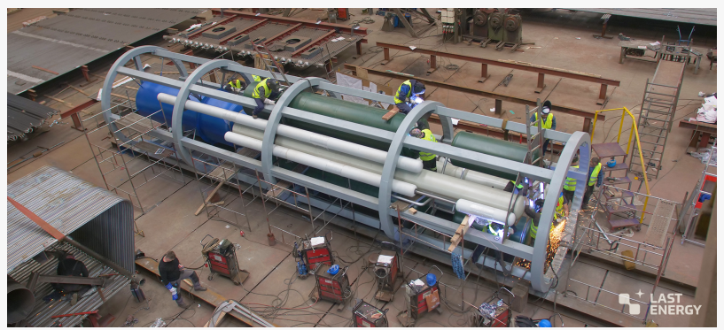
Factory fabrication of a Last Energy demonstration module in Poland in 2023
