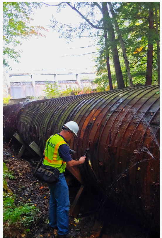
Jackman Penstock Replacement Project located in Hillsboro, New Hampshire.
