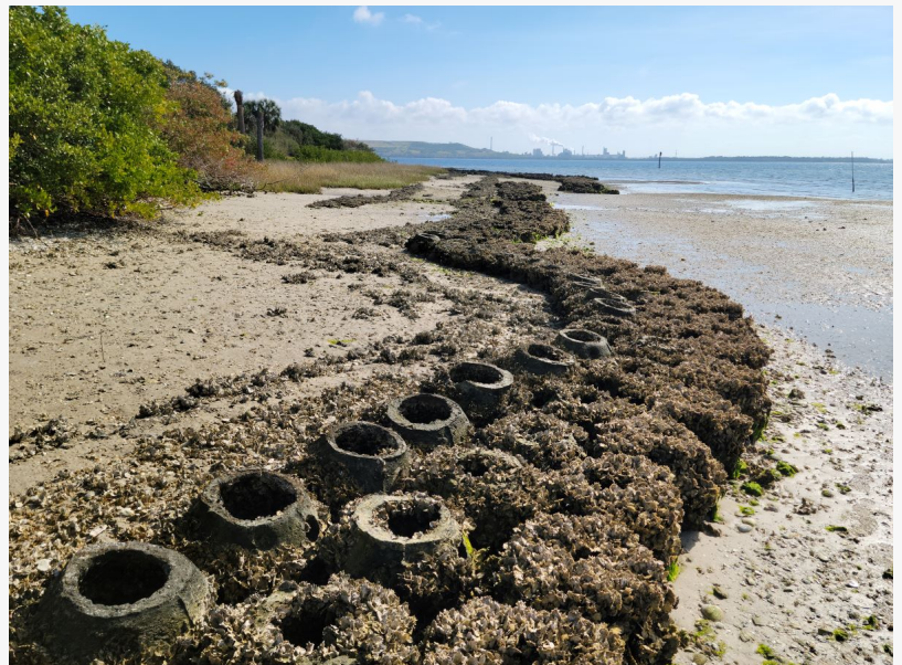
At low tide, a living shoreline installed by Tampa Bay Watch reveals new oyster growth on marine-safe oyster reef balls. These ORBs serve as barriers against harmful wave action and provide habitats for hundreds of oysters and other marine invertebrates.
