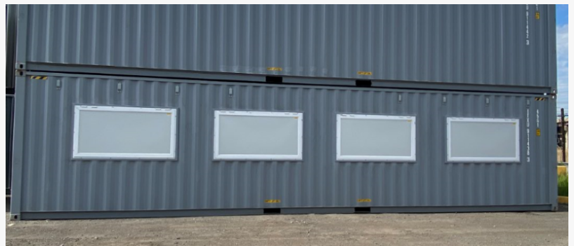
Shipping containers being converted into modern, eco-friendly homes
