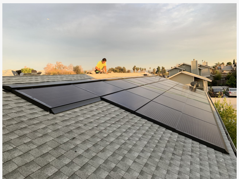
Rooftop Solar Panel Installation
