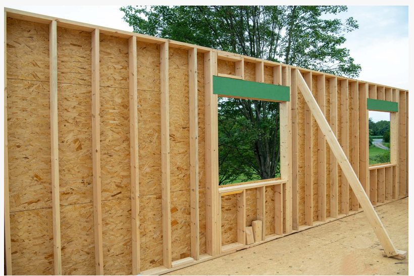
ADU built to last from the ground up
