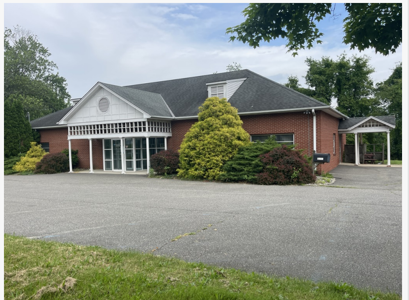
Former Medical Office Bldg, Branchburg Twp, NJ
