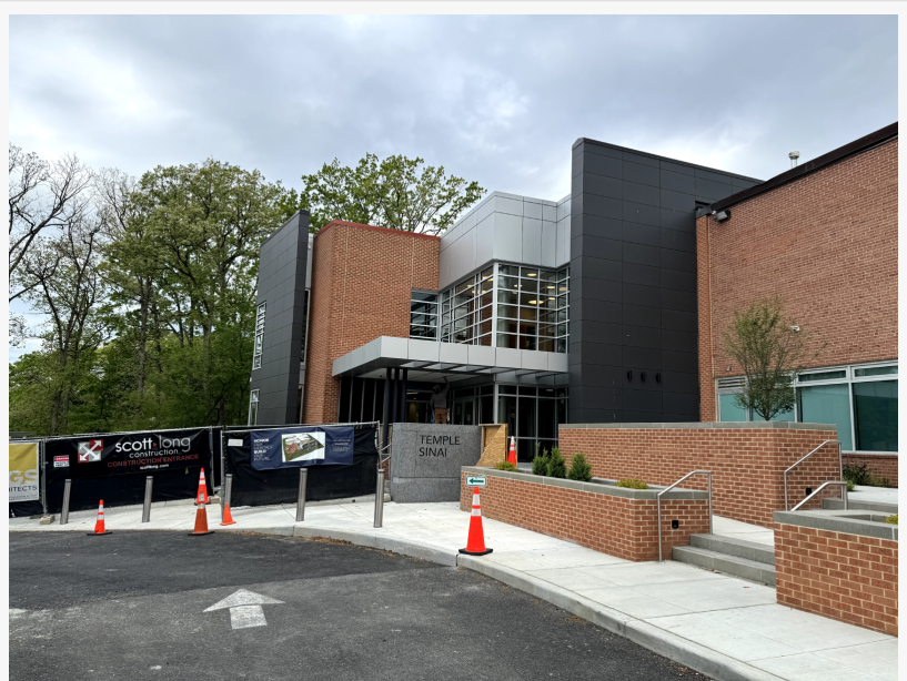
Metro DC commercial construction Temple, Sinai rain screen
