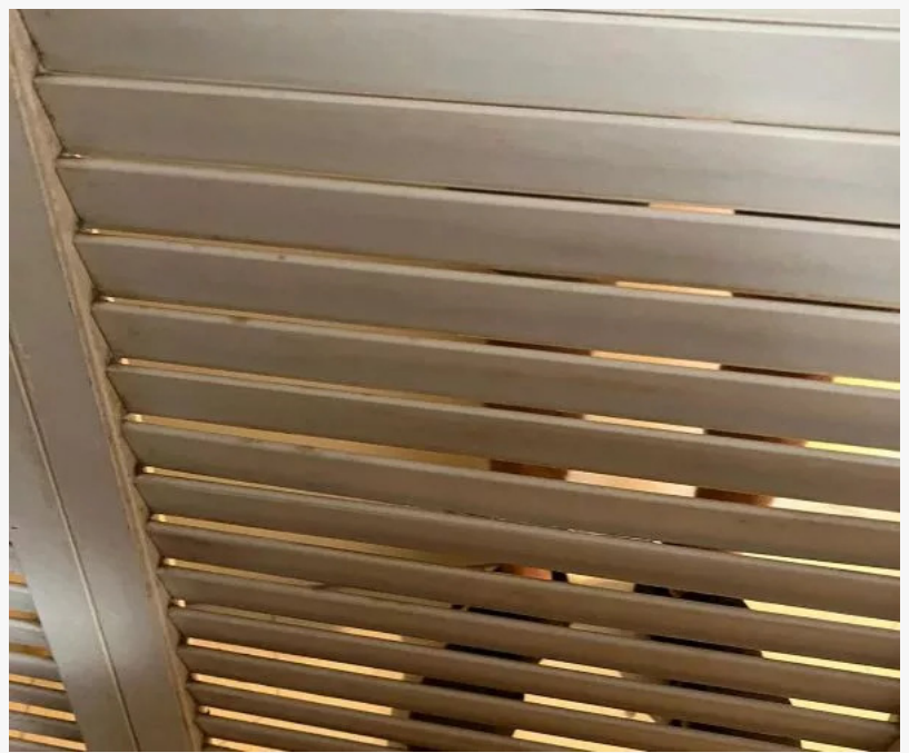
clean Qaulity Air - Air Duct Cleaning
