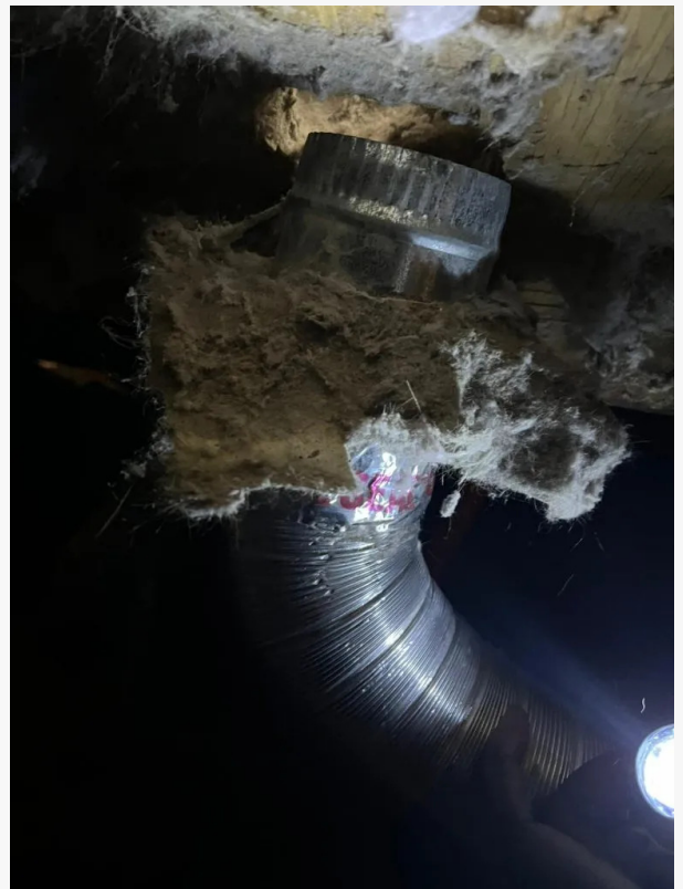
Commercial Air Duct Cleaning Services
