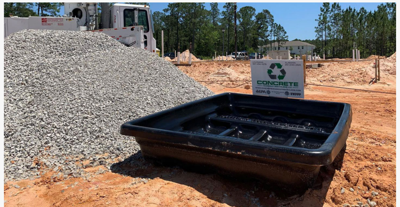
Concrete Washout Basin
