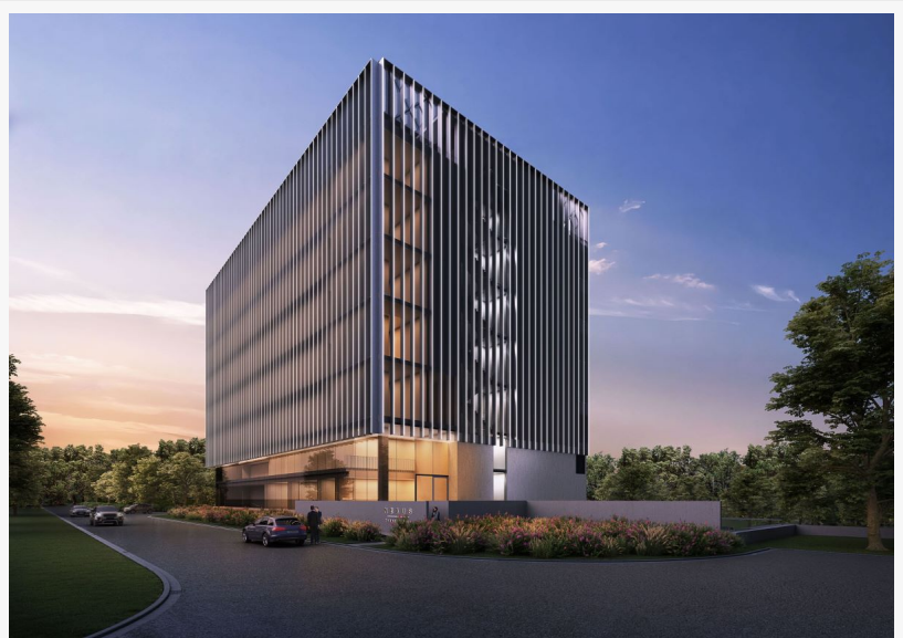
Penta Infra's new 7.2 MW data center in Brussels
