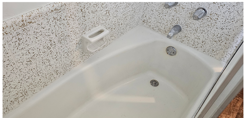
Hollywood tile restoration and regrouting
