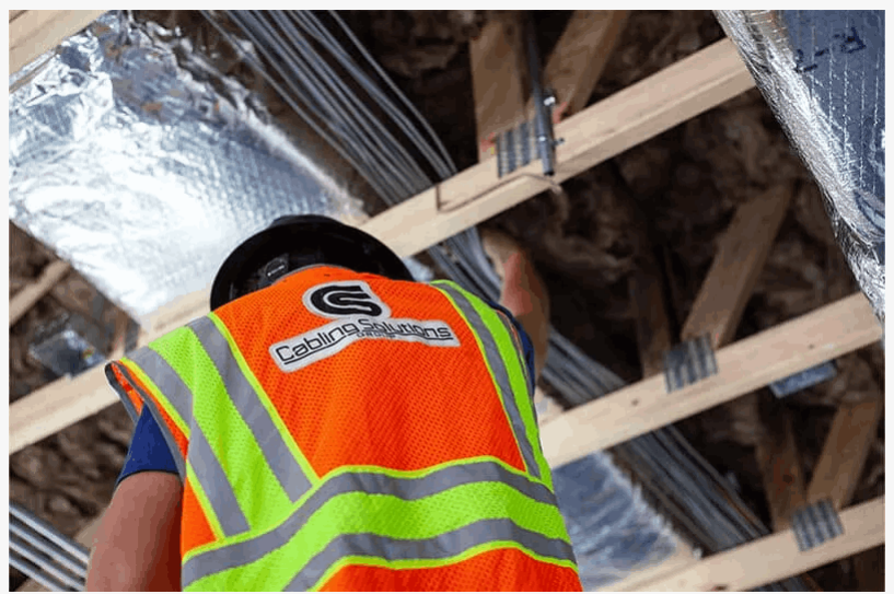
Cabling Solutions Group Installing Structured Cabling
