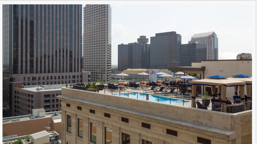
Rooftop aerial view
