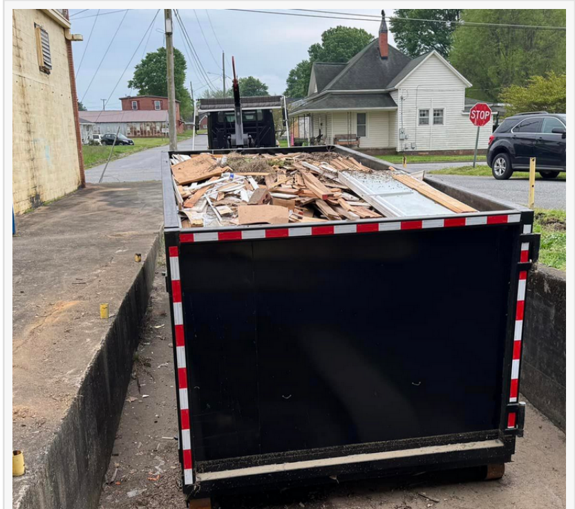
Construction debris piled high in a dumpster on an urban street.
