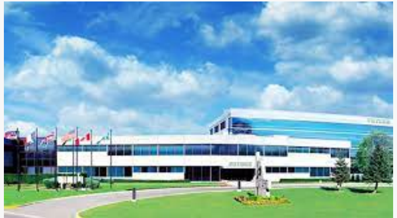
Future Electronics Headquarters
