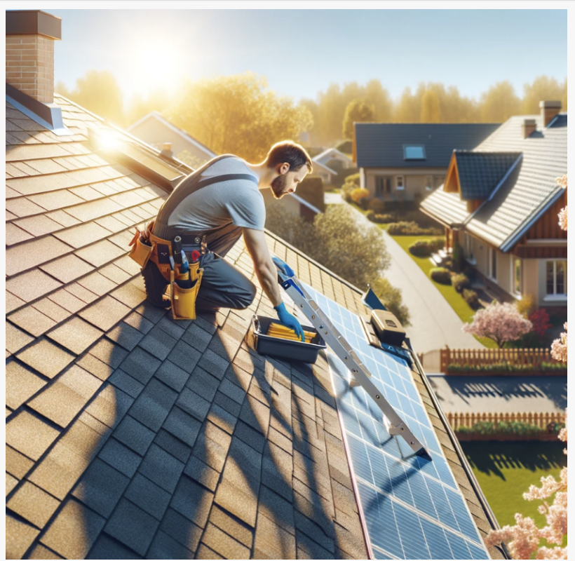
Intelligent Design Air Conditioning, Plumbing, Solar, & Electric Solar Installation in Tucson
