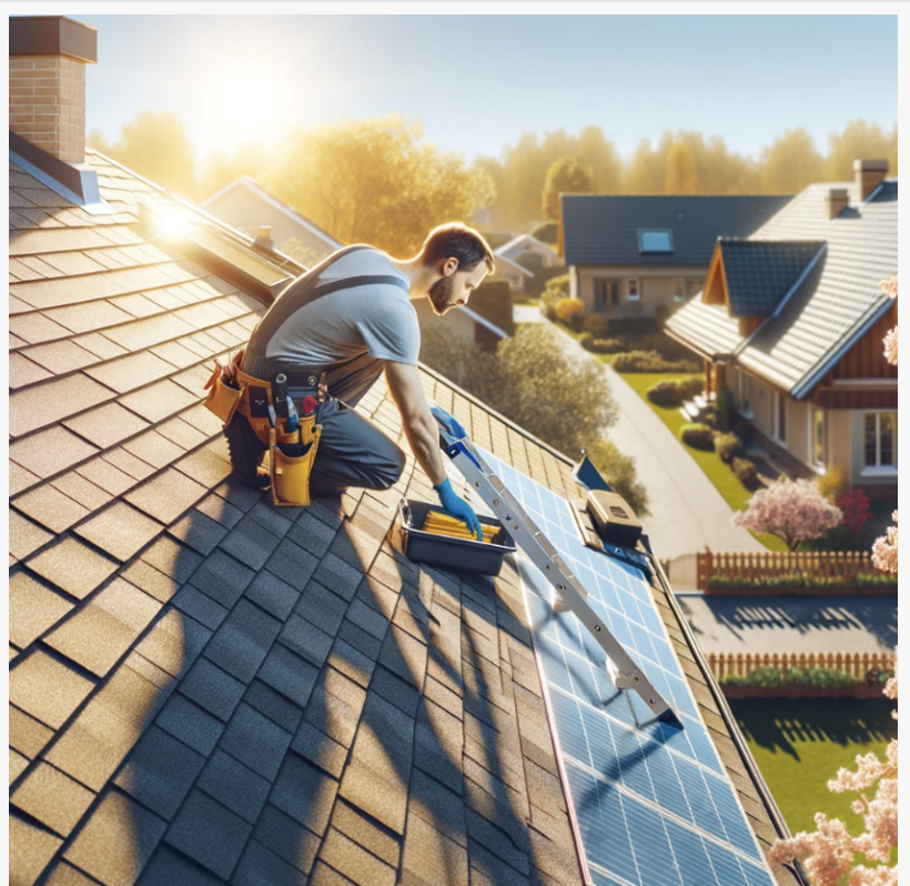
Intelligent Design Air Conditioning, Plumbing, Solar, & Electric Solar Installation in Tucson
