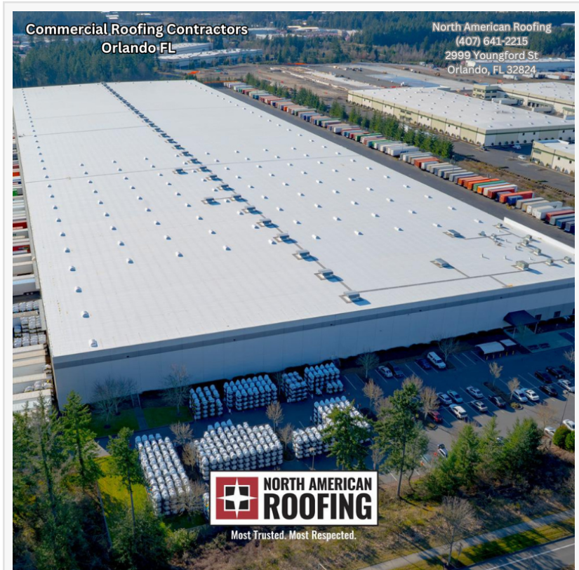
North American Roofing: 45 Years as Trusted Commercial Roofing Contractors in Orlando FL.
