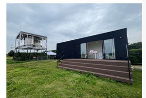
A wind power generator connected to a house
