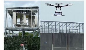
Vertical wind power generators A delivery drone for emergency use
