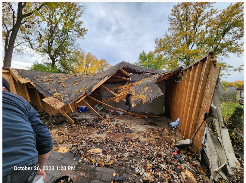
Garage Demolition (before DemoPro)
