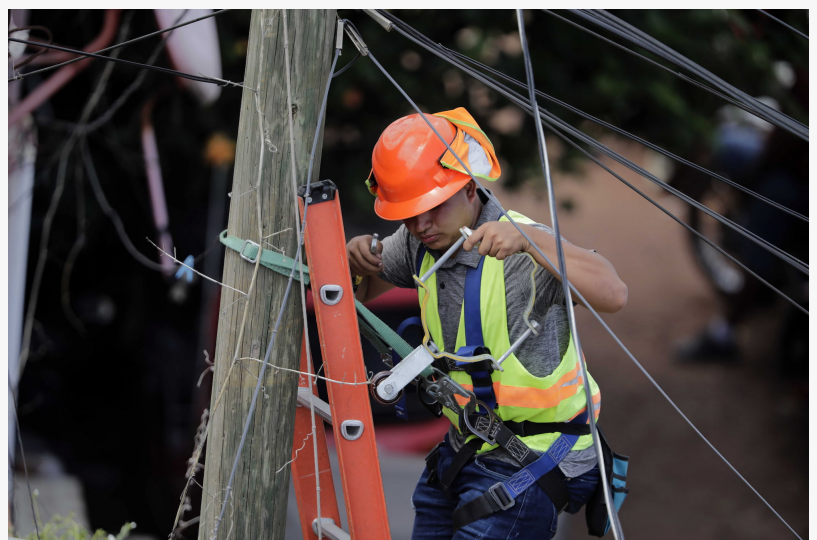
Supply of aluminum overhead cable construction for Honduras
