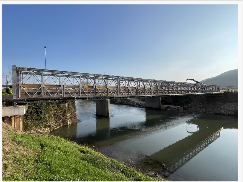
Acrow box bridge in Vicenza
