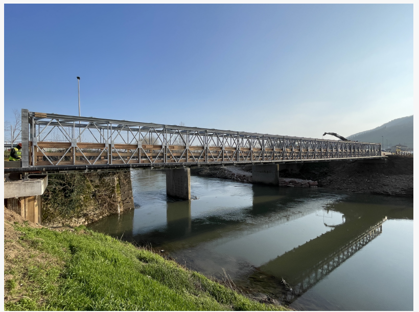
Acrow box bridge in Vicenza
