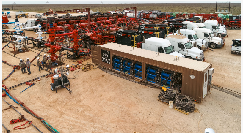
Comanche Gas Distribution on location in Permian Basin
