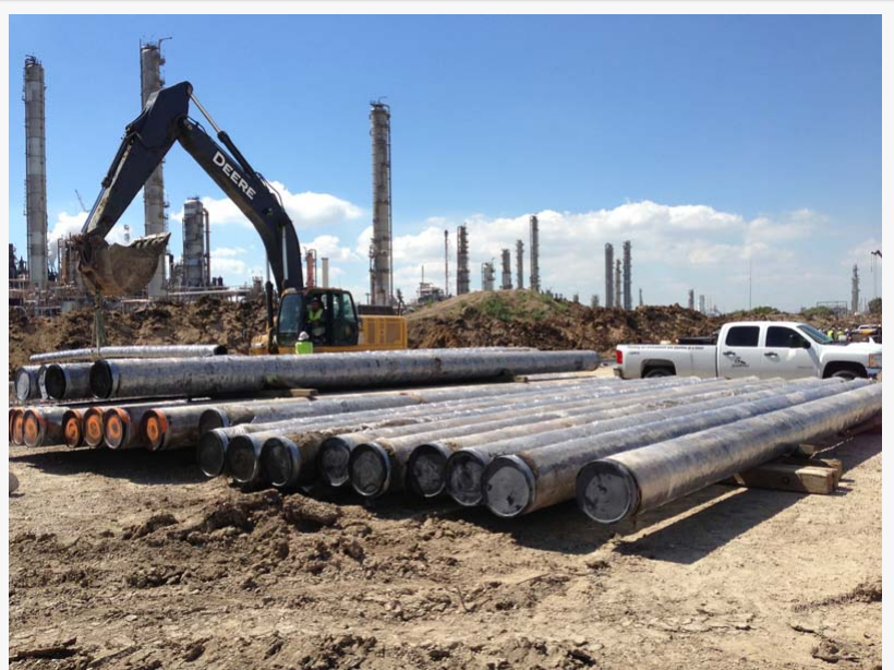
Southwest Pipe Services Inc Environmental Services for Pipeline Abatement
