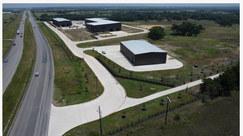
CRA opens new manufacturing facility in Brenham, Texas
