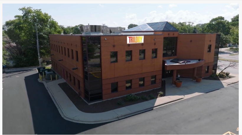
Trilogy's 24,000-square-foot wellness center at 8541 S. State Street.
