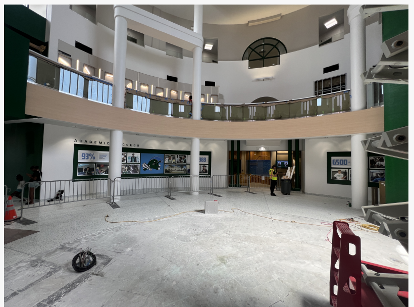
After Photo of Di NOC wrap install at Tulane University
