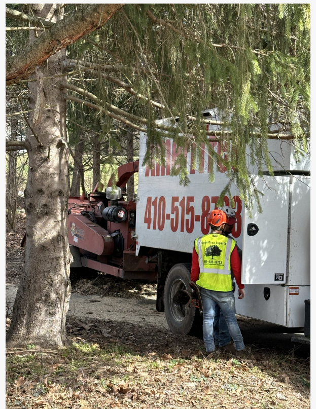
AmeriTree Experts Truck and Crew Working on Tree Removal
