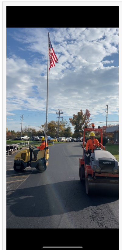
Montgomery County, MD Asphalt Driveway Paving
