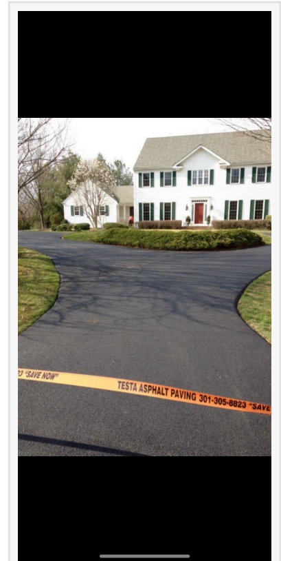
Frederick County, MD Asphalt Driveway Paving
