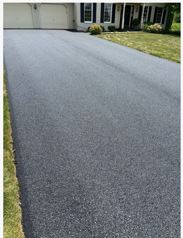
Asphalt Driveway Paving in Reading, PA
