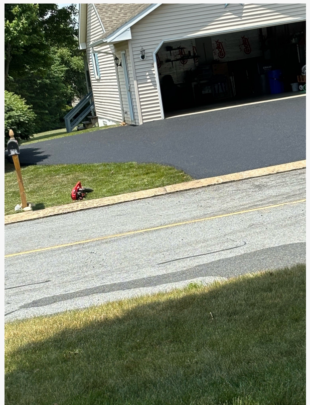
Asphalt Driveway Paving in Lancaster, PA
