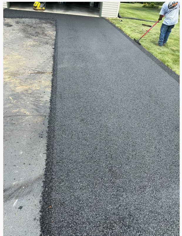
Asphalt Driveway Paving in the Reading, PA and Lancaster, PA Region
