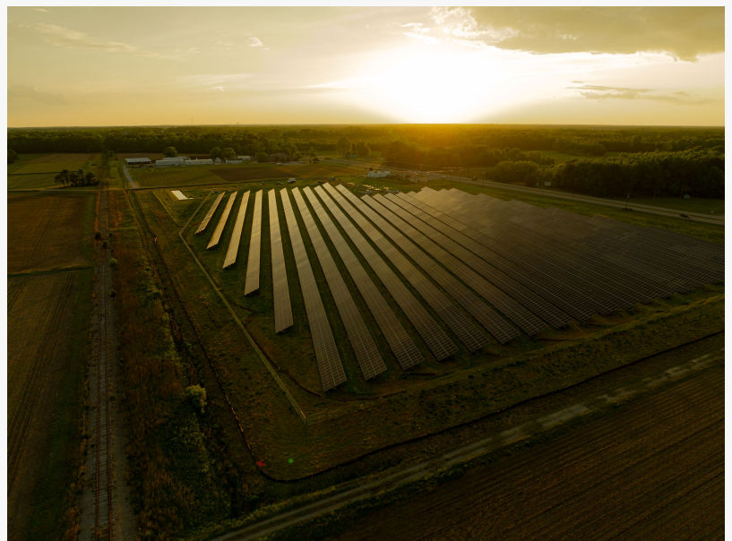
Community solar project by Dimension Energy (Suffolk, VA)
