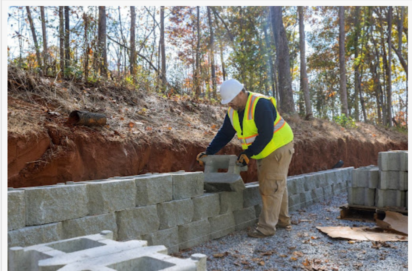
A hardscaping contractor in full safety gear is installing a retaining concrete block wall on a new property surrounded by tall trees, showcasing professional retaining wall services.
