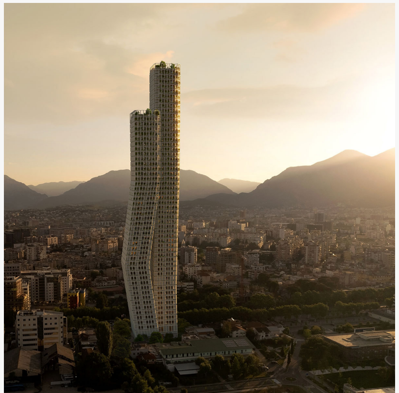
Bond Tower, By OODA, Aerial View
