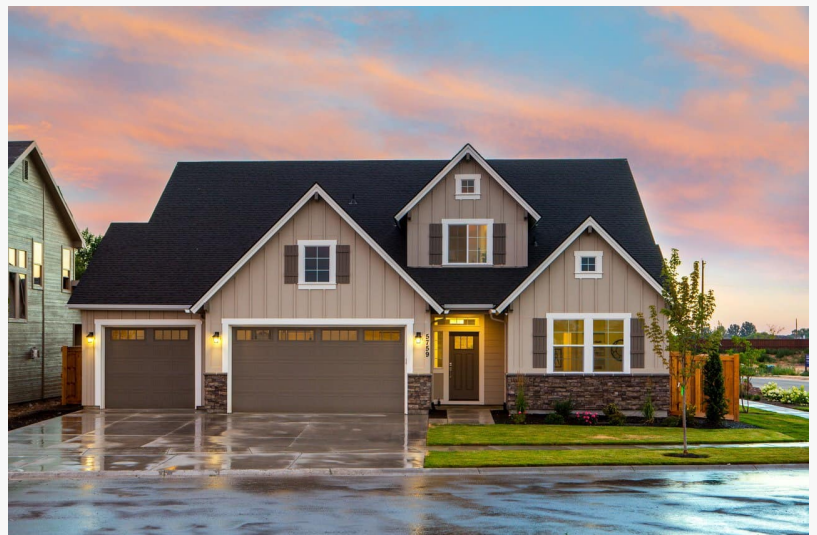
Roofing Company in DeBary
