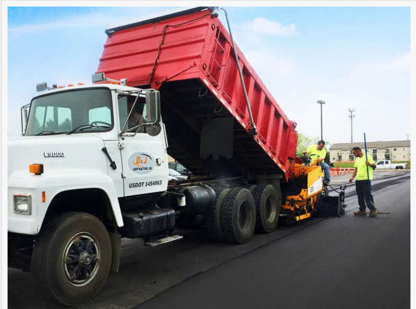
D&J Contracting, Inc - Commercial Asphalt Maintenance & Installation
