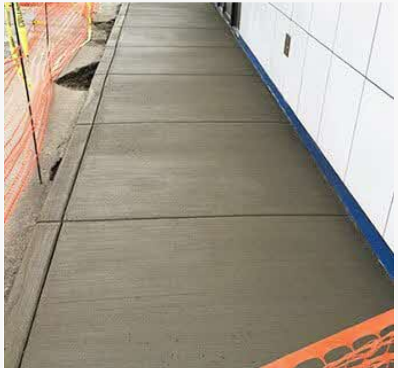
Commercial Concrete Repair & Installation
