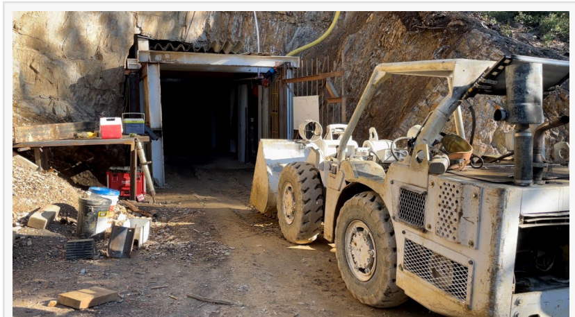
Mt. Vernon Mine Portal
