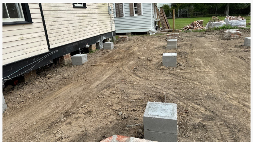
Baton Rouge Foundation Repair
