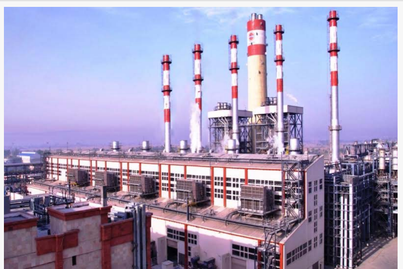
Captive Power Plant
