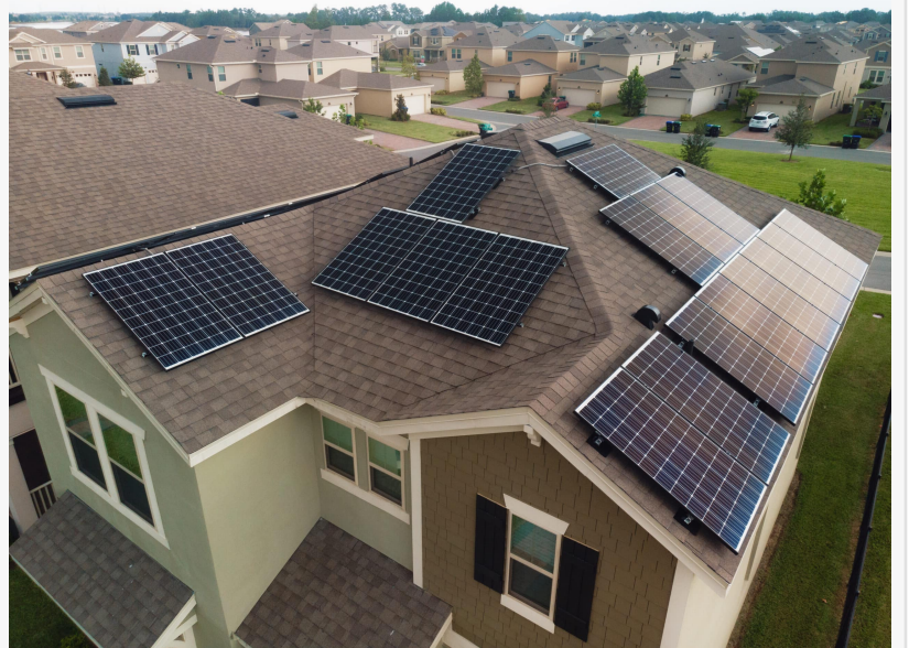
Orlando solar panel installers
