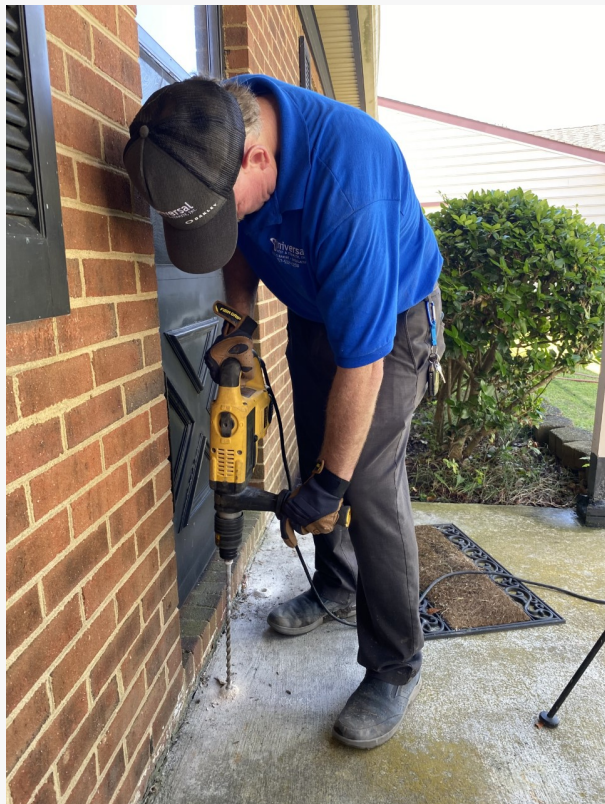
Termite treatment chesapeake virginia
