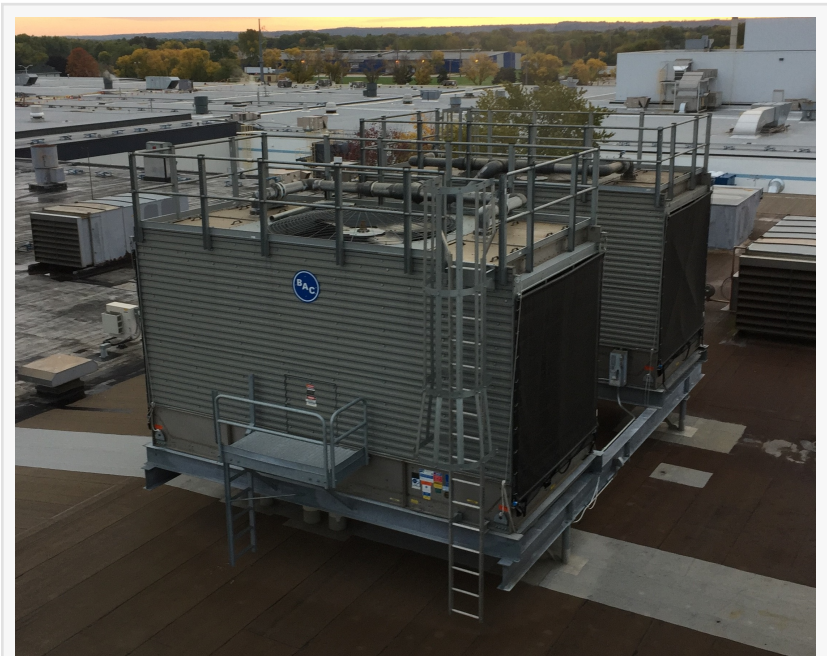
Industrial Cooling Towers Being Installed
