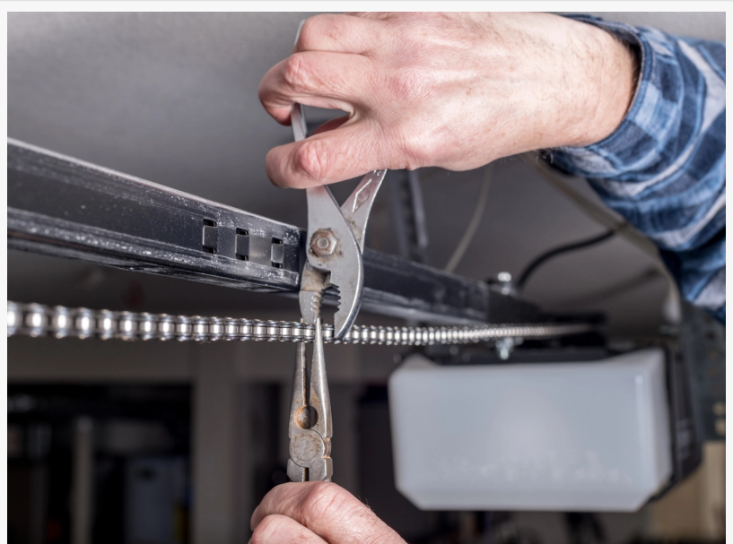
Fast Garage Door Spring Repair
